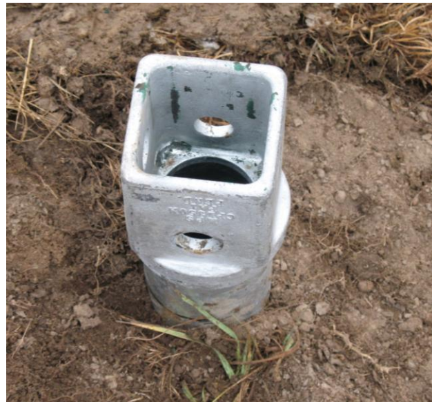
Pipe pile and coupling system remains undamaged during installation
