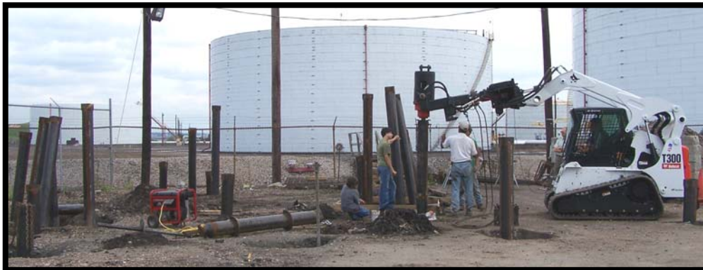
Lightweight and maneuverable equipment was used to installed the helical piles
