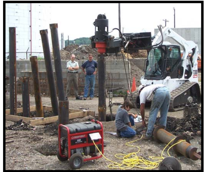
Lightweight and maneuverable equipment was used to installed the helical piles
