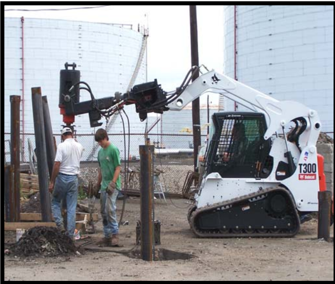
Lightweight and maneuverable equipment was used to installed the helical piles
