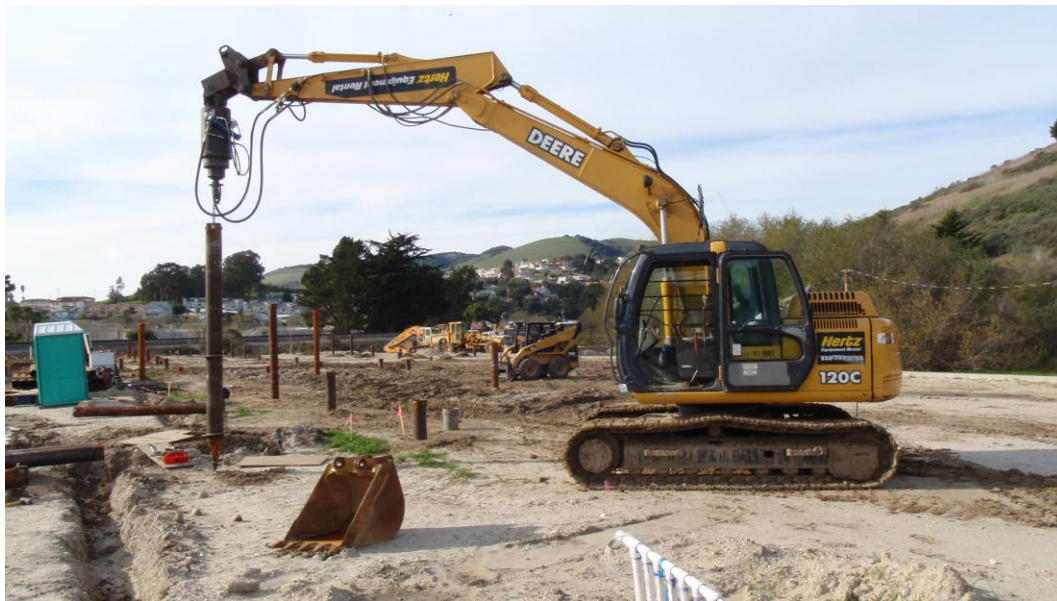
New construction with P8
